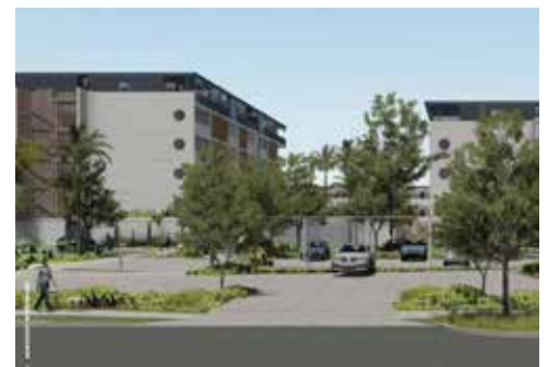
General View of Development
