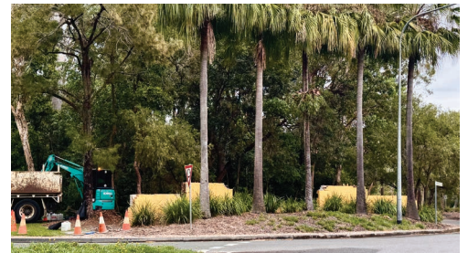
Wall being demolished this week
